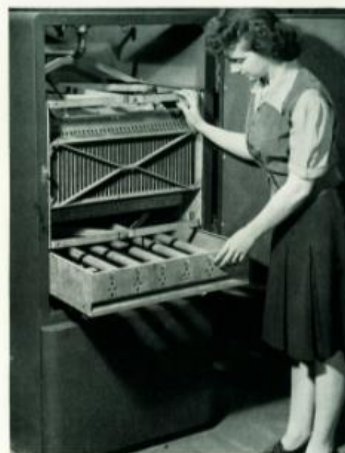
An Electronic Housemaid Guards Your Home from Dirt If windows are kept closed, and air fed into the house through a central ventilating or heating system, this Proscopion eliminates sweeping. As air rushes through the "blower" open at the bottom, dust particles are electrified by tungsten wires, then fished out of the air stream by charged metal plates.
