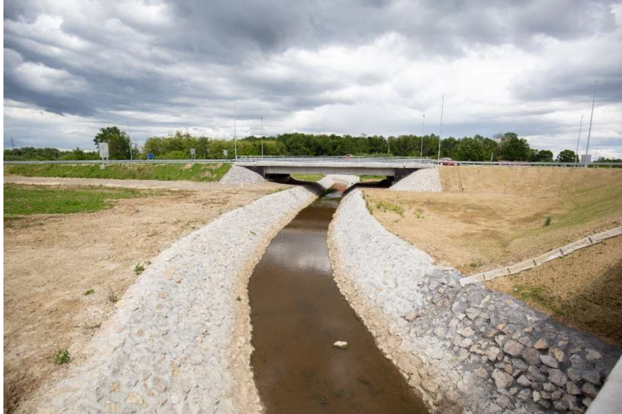
Figure 6 – Intensive structural measure - Example of flow acceleration (floodway).
