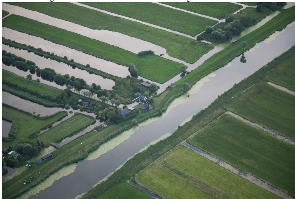
Figure 5 – Extensive structural measure: Vegetation cover control.
